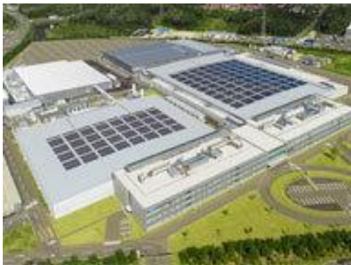
Fig.3 View of Tokyo Electron Miyagi
